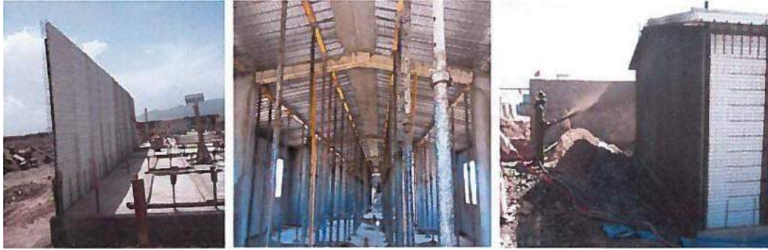
Figure 1.3. Construction with 3D panels; (a) erection Of wall panels; (b) slab panel; (c) shotcreting. after Mashal (2011)
