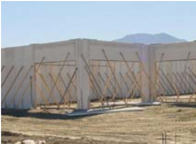
Braces are used to support panels during construction
